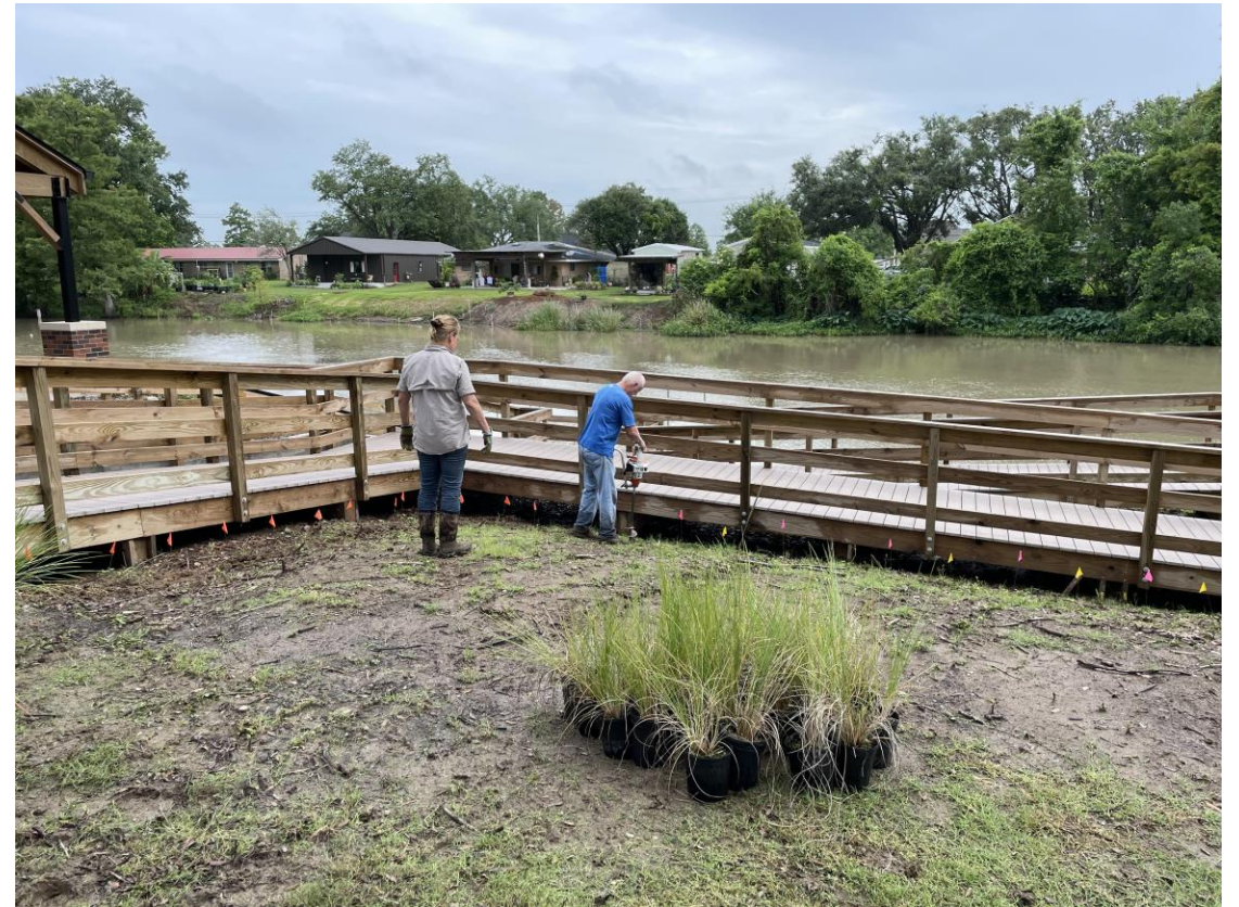
Bayou-Side Pier Planting
